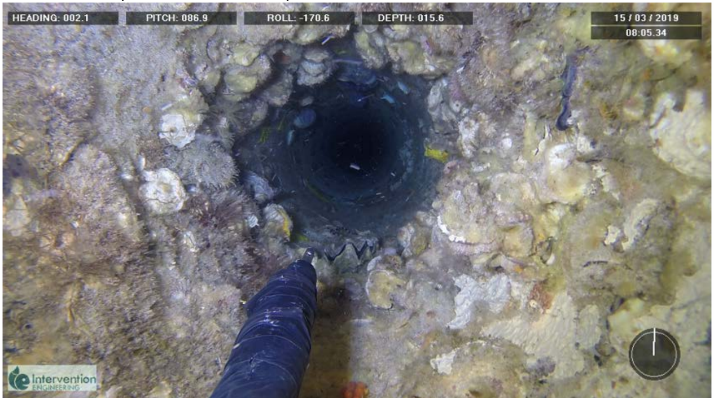
Prior to Cleaning (13m long tube)
