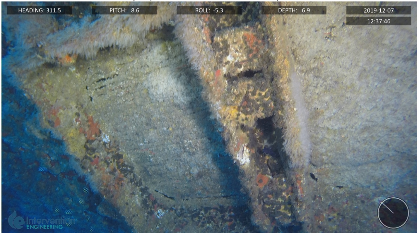
Before cleaning and fitting of water blaster showing almost total coverage of soft growth
