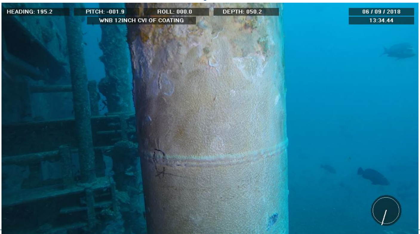
Cleaned down the good coating prior to scanning and clamp installation
