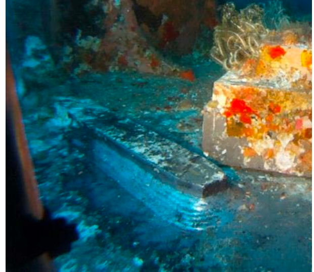
After Cleaning to expose Weld
