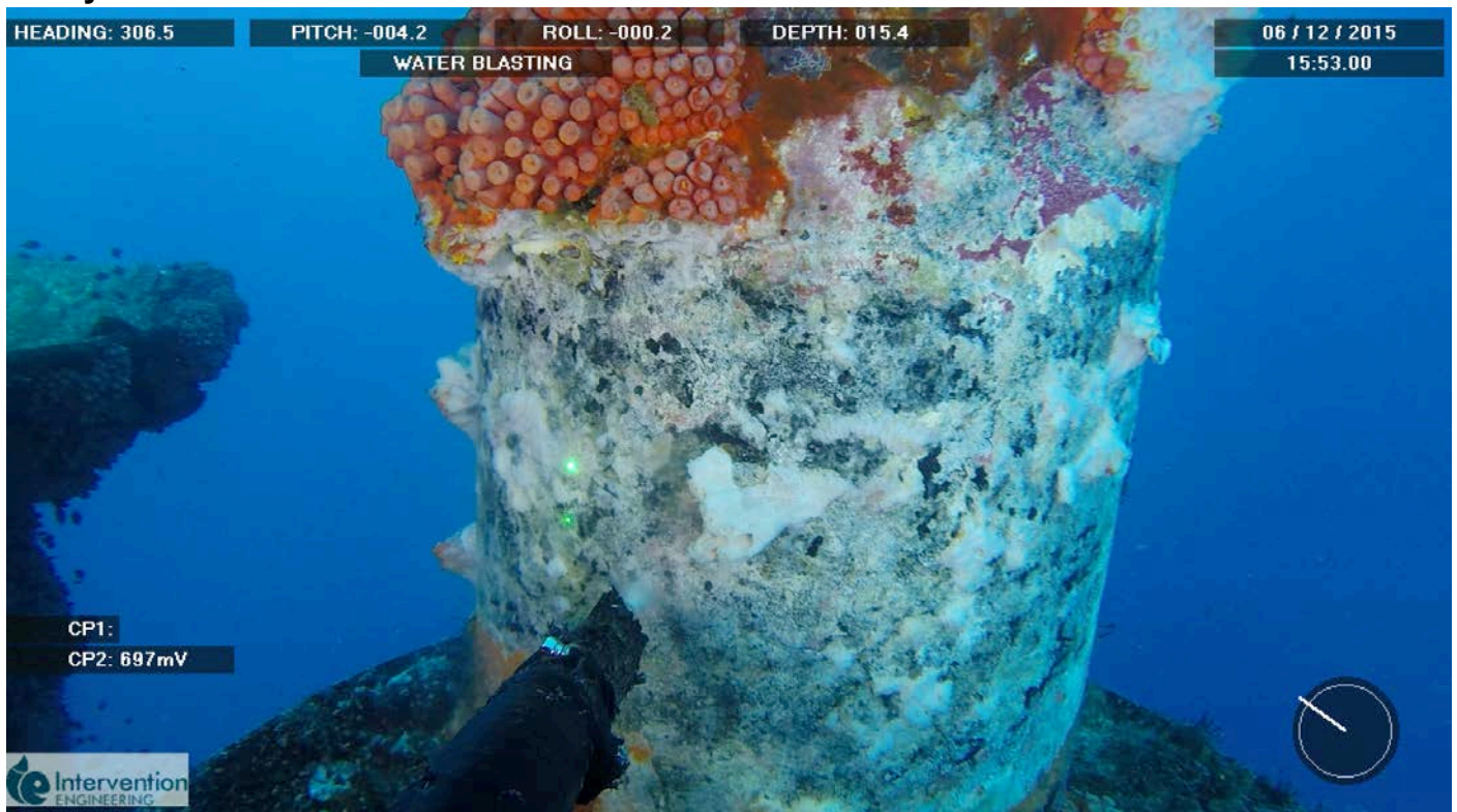
Hacking through the heavy coral – the nozzle is 60mm wide, so coral is well over 100mm
